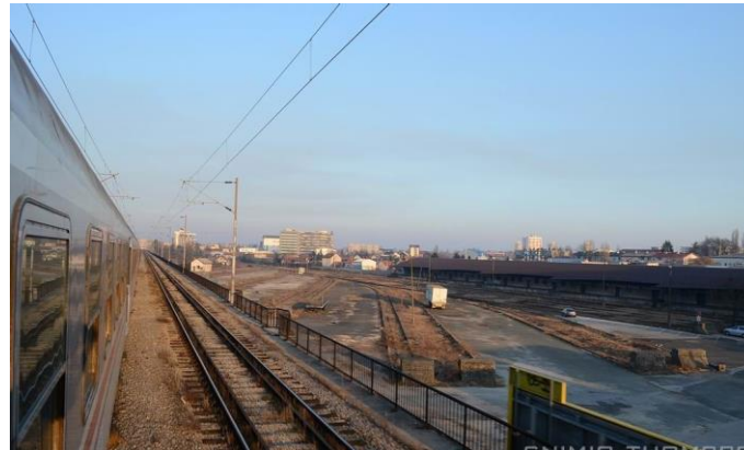
Eastern Railway Station
